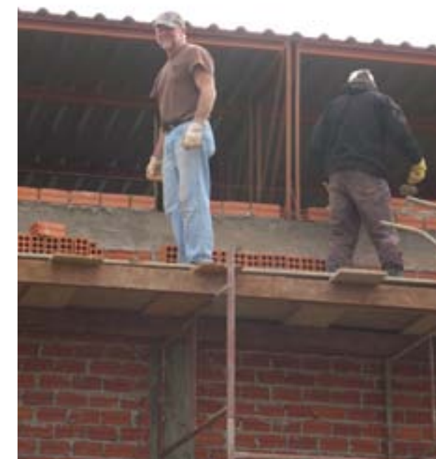
Bobby Wacaser helps with the construction
